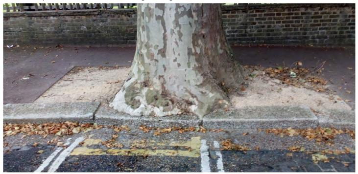
Increased tree pit size, infilled with self-binding gravel <sup>249</sup> Tree Policy 2020- 2030 These will be considered on a case by case basis and include:
